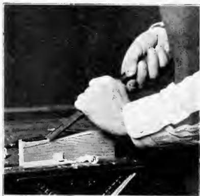
Fig. 69. Paring With a Chisel.
