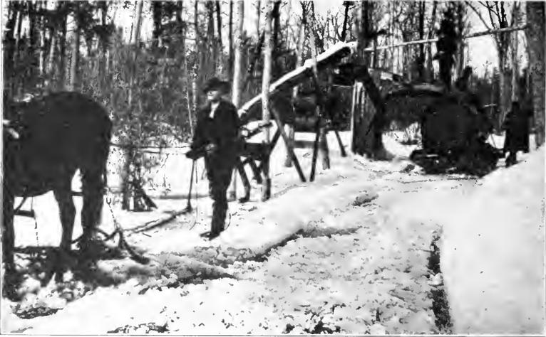
Fig. 10. Making an Ice Road by Flooding.
