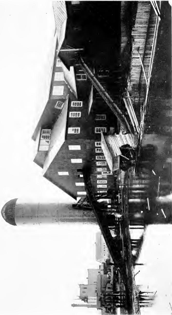
Fig. 37. Two-Story Mill at Virginia, Minnesota, Showing Jack-Ladders and Consmmer.
