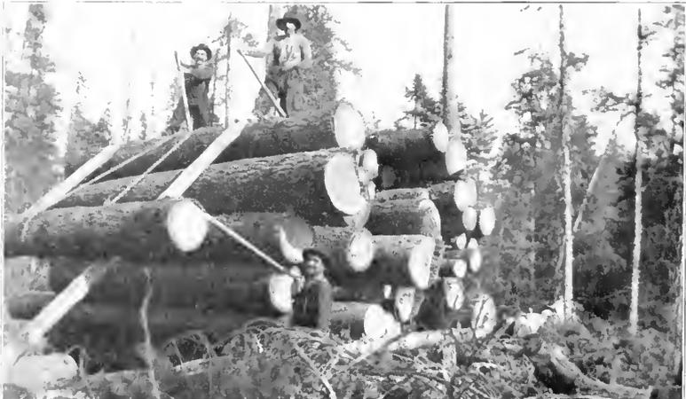
Fig. 11. Decking Logs on Skidway.
