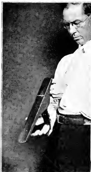
Fig. 102 Sighting Along the Sole of Jack-Plane
