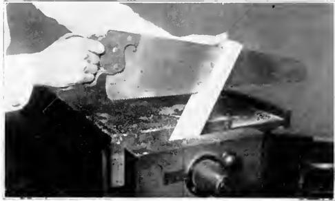
Fig. 89. Rip-sawing with Wood Held in Bench-Vise.
