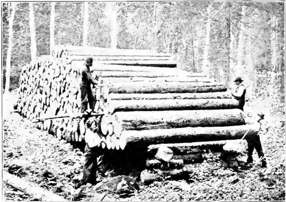
Fig. 9. "Scaling" Logs on the Skids.
