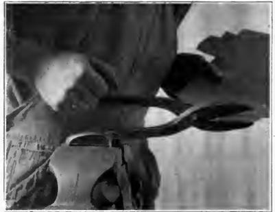
Fig. 105. Cutting copper with snips.
