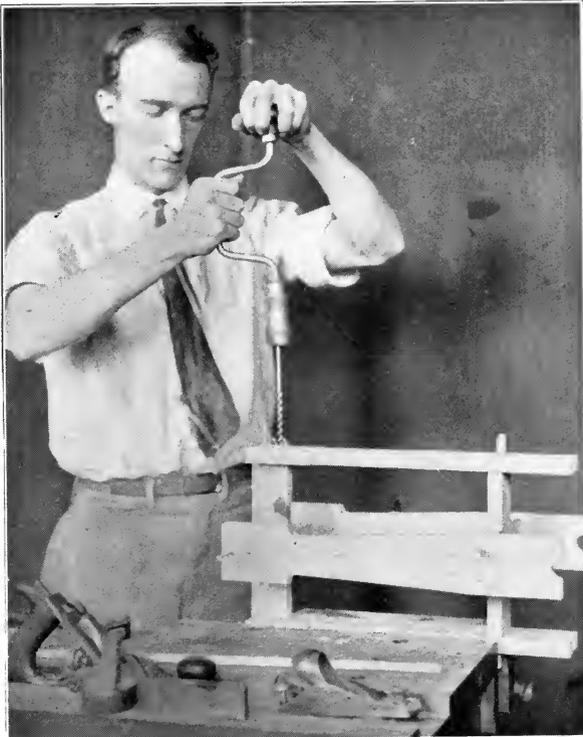
Fig. 137. Boring the holes for the dowels.
