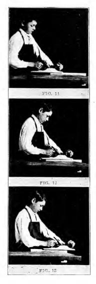
bottom of the tool may be in the same plane as the surface of the board you are handling.
