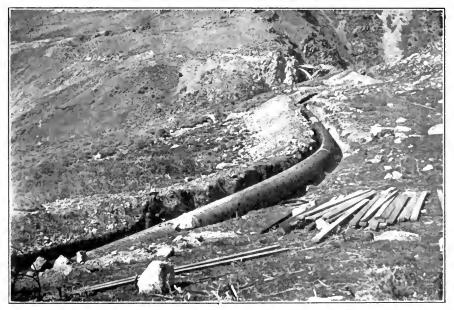
FIG. B.-36-inch wooden stave continuous pipe.
