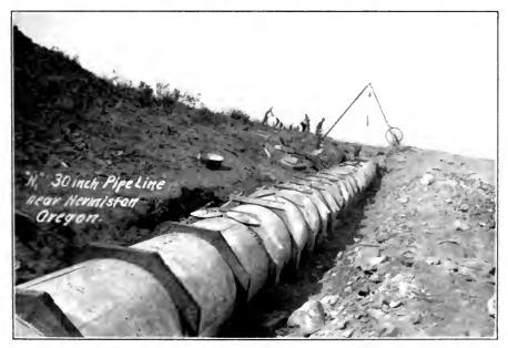
FIG. B.—Cast collars on 30-inch reinforced concrete pipe. Umatilla Project, Ore. (Facing page 315)
