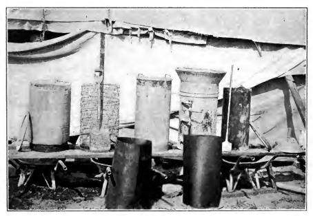
FIG. B.—Moulds for making small size reinforced concrete pipe. Tieton Project, Wash. (Facing page 314)
