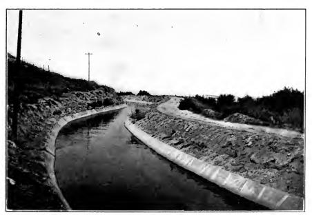
FIG. B .- Concrete-lined eanal near Riverside, Calif.
