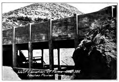
FIG. B.-Reinforced concrete flume. Naches Power Canal, Wash.
