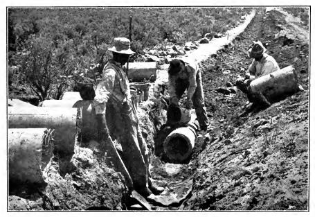
FIG. D.-Laying and joining reinforced concrete pipe. Tieton Project, Wash.
