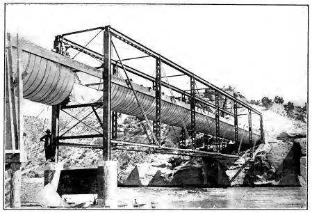
F1G. D.—Lennon steel flume, 9 feet diameter on 110-foot span steel bridge over Las Animas River, Cedar Hill, N. Mex., for Aztee Irrigation Co.
