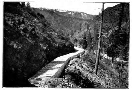
FIG. C.—Tieton diversion canal, formed with reinforced concrete shapes. Tieton Project, Wash.
