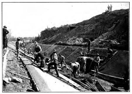
FIG. D.-Placing concrete lining. Ridenbaugh Canal, Idaho.
