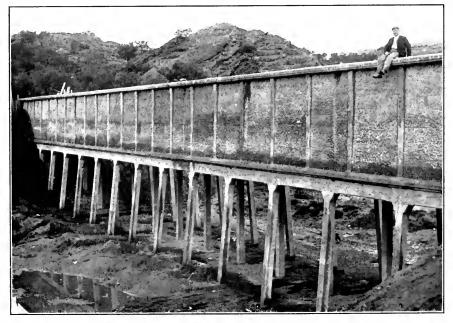
FIG. D.-Reinforced concrete flume. Faleva Flume, Spain.
