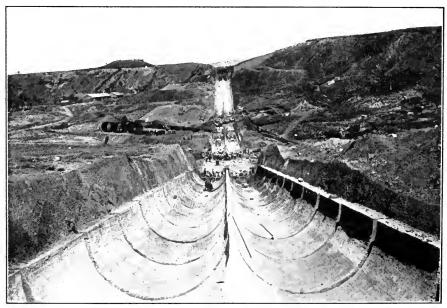
FIG. D.—Cradles of lean concrete to support reinforced concrete pipes of Sosa Siphon, Spain.
