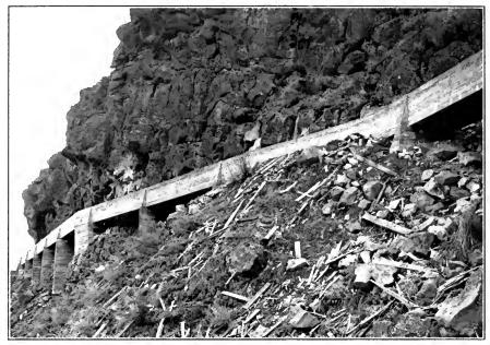
FIG. C.-Reinforced concrete flume. Naches Power Co., Wash.
