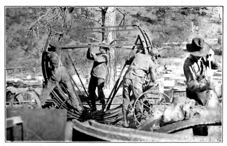
FIG. B.-Adjusting metal moulds. Tieton Project, Wash.
