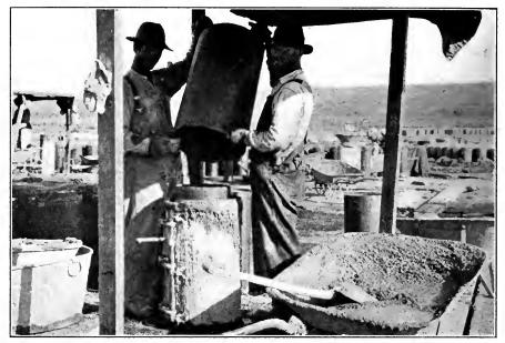
FIG. C.—Placing reinforcement eage, surrounded with tarred paper cylinder, in moulds. Tieton Project, Wash.
