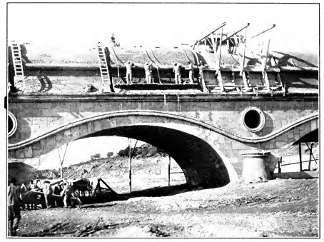
${\tt Fig.\,C.-Construction\,of\,concrete\,shell\,around\,steel\,tubes\,on\,bridge.}\ Sosa\,Siphon, {\tt Spain.}$
