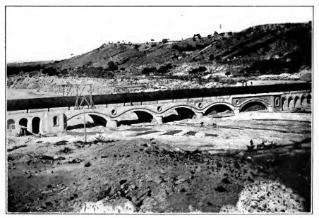
FIG. B.—Steel tubes in position on Sosa River Bridge, Spain. (Facing page 334)
