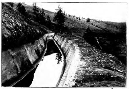
FIG. D.—Completed concrete-lined eanal. Kamloops Fruitlands Irrigation & Power Co., B. C.
