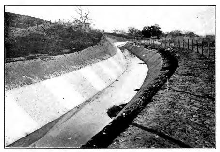
FIG. D,-Concrete-lined canal. Yolo Water and Power Co., Irrigation System, Calif.
