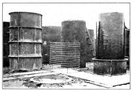
FIG. B.—Moulds for casting 47-in. reinforced concrete pipe. Umatilla Project, Ore. (Facing page 304)
