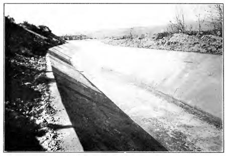
FIG. C.-Concrete-lined canal. Ridenbaugh Canal, Idaho.
