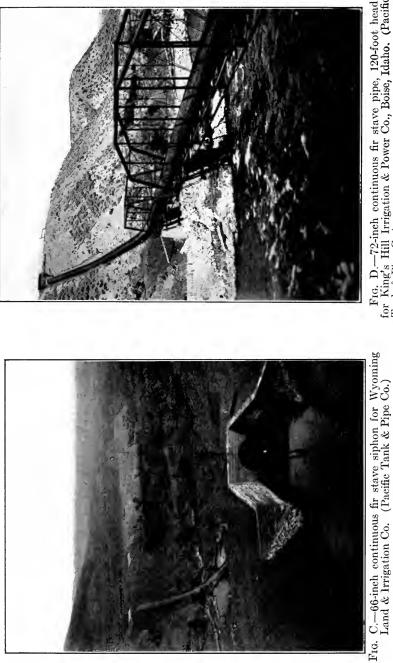
FIG. D.—72-inch continuous fir stave pipe, 120-foot head, for King's Hill Irrigation & Power Co., Boise, Idaho. (Pacific Tank & Pipe Co.)
