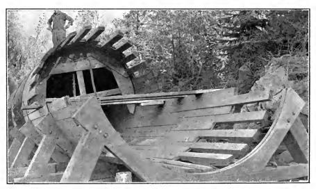
FIG. D.--Construction of wooden stave pipe on cradles.
