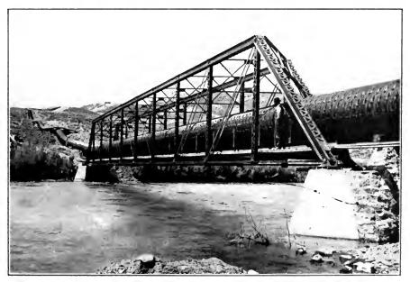
F1G. B.—60-inch continuous wooden stave pipe on bridge over Bear River, Oneida Irrigation District, Idaho. 300-foot head,  $\frac{3}{4}$ -inch bands,  $\frac{5}{5}$ -inch center to center. (Pacific Tank & Pipe Co.)
