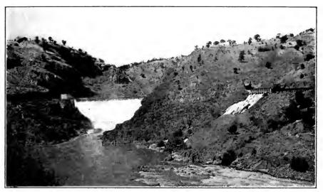
FIG. A.—Diversion dam and headworks for Modesto and Turlock Irrigation Systems, Calif. Diversion dam is about 130 feet high.
