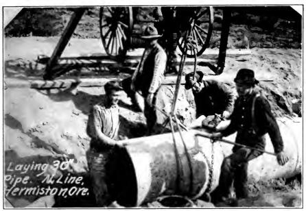
FIG. A .- Laying and joining 30-inch reinforced concrete pipe. Uinatilla Project, Ore.
