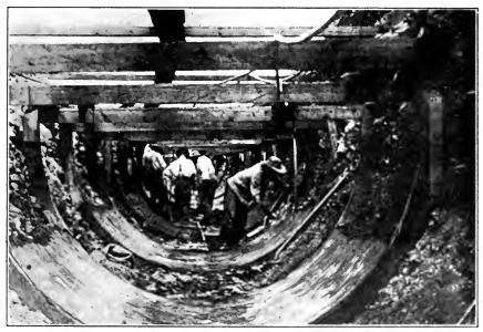
FIG. B.—Constructing semicircular concrete lining. Umatilla Project, Ore. (Facing page 168)
