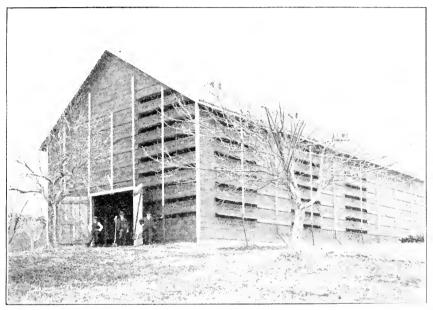
FIG. 1.—Type of barn used in northern eigar-tobacco districts, showing the arrangement of horizontal ventilators.
