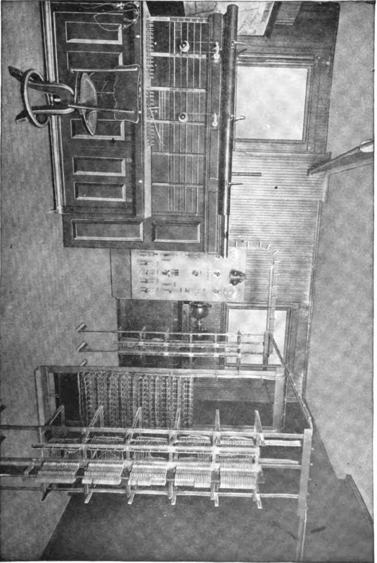
*Fig. 3.—General Relation of Switchboard and Distributing Board.*
