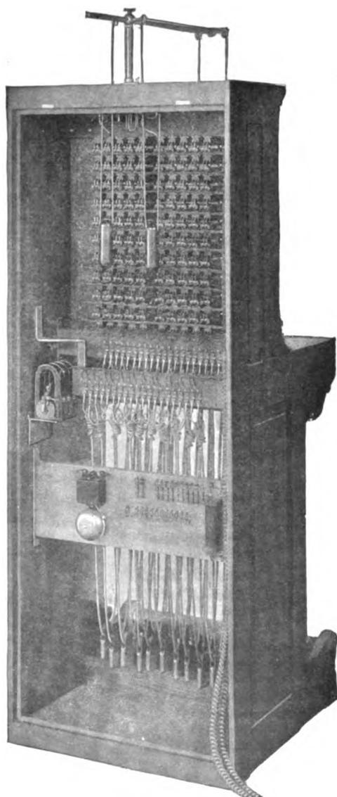
*Fig. 32. — Rear View of Small Switchboard.*
