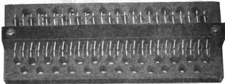
Fig. 13.—Street Cable Clips Distributing Board.
