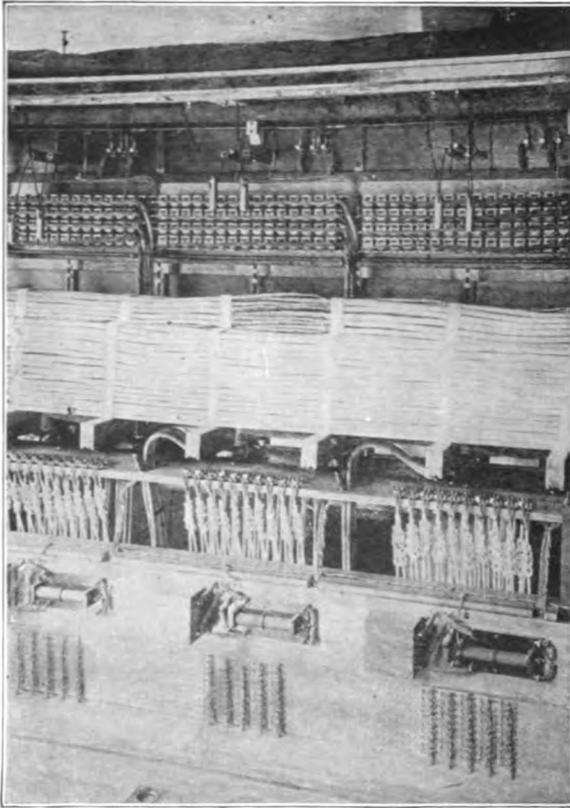
*Fig. 68.—Rear View of a Branch Terminal Board.*
