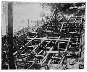
FIG. 251.-Stationary pneumatic caisson.
