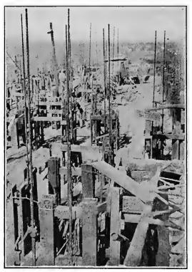
FIG. 215.-Attachment of jacks to rods.
