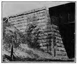
FIG. 128.-Masonry U-abutment.
