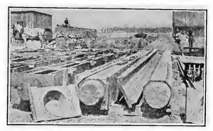
FIG. 239.-Precast concrete piles.
