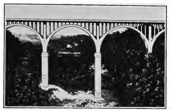
FIG. 64.—Arch with thin piers at Akron, Ohio.
