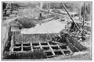
FIG. 244.-Telescoped sheet piling coffer-dam.
