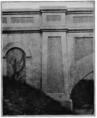
Fig. 148.—Paneled bridge abutment.
