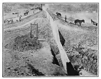
FIG. 101.-Earth fill dam with core wall.
