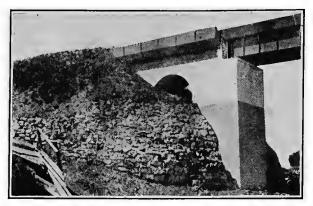
FIG. 132.-U-abutment with open side walls.
