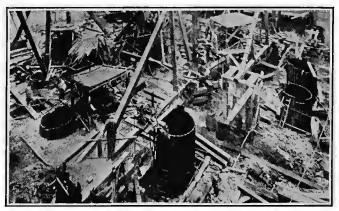
FIG. 231.-Open well foundation.
