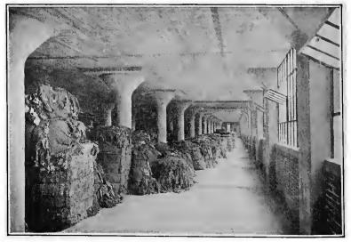
FIG. 37.-Flat slab warehouse floor with drop panels.
