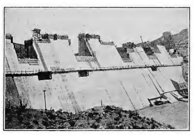
FIG. 93.-Elephant Butte dam during construction.
