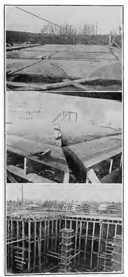
FIG. 220.—Forms for groined arches at Whitinsville, Mass. Showing method of construction.
