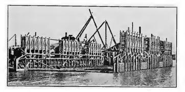
FIG. 263.—Pontoon for launching a caisson.
