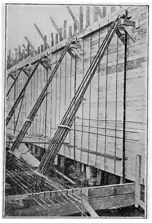
FIG. 116.—Reinforcement in counterfort retaining wall.
