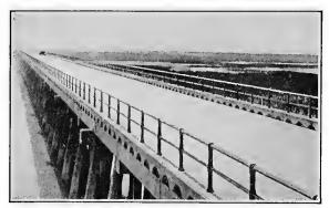
FIG. 160.—Reinforced concrete highway trestle.
