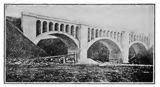
FIG. 67.-Vermillion River bridge showing spandrel arches.
