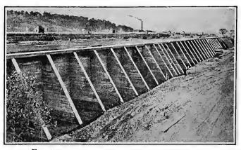
FIG. 115.-Rear view of counterfort retaining wall.
