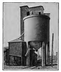
FIG. 194.—A reinforced concrete sand bin.
