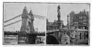
FIG. 150.—Architectural treatment of bridge piers. Hammersmith Bridge, London, and bridge over Amstel, Amsterdam.
