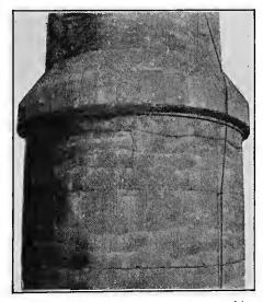
FIG. 198.-Temperature cracks in a concrete chimney. •
