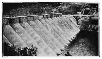
FIG. 97A.-Lake Hodges multiple arch dam. Upstream face.
