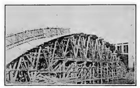
FIG. 217.—Pile bents used as centering.
