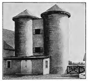
FIG. 195.-Reinforced concrete twin silos.
