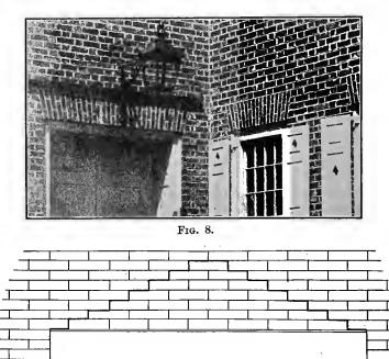
FIG. 9.—Masonry supported by a lintel.
