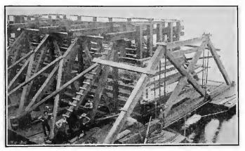
FIG. 261.-Caisson supported by barges.
