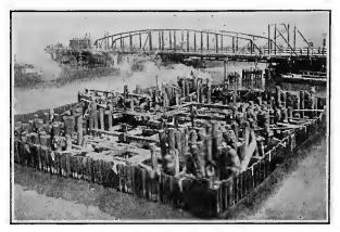
FIG. 233 .- Pile foundation, 92nd St. bridge, Chicago.
