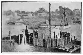
FIG. 243.-Steel sheet piling coffer-dam.
