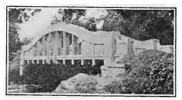
FIG. 166.—Reinforced concrete truss bridge.
