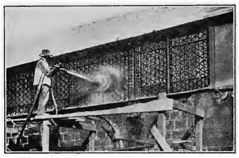
FIG. 22.-Covering a steel girder with concrete by means of a "cement gun."
