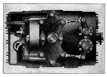
FIG. 198. — AIR CYLINDER WITH MECHANICAL DISCHARGE VALVE.
