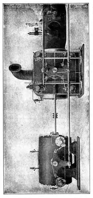
FIG. 200. — CROSS-COMPOUND TWO-STAGE AIR COMPRESSOR, SHOWING LOW-PRESSURE CYLINDER AND VALVE GEAR.
