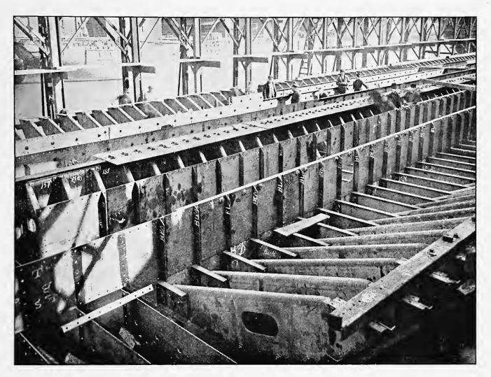
STUART'S CHANNEL SYSTEM OF CONSTRUCTION .- Showing keel, keelsons, intercostals and floors.
