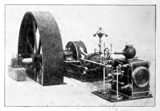
Fig. 26. Simple Corliss Engine, Showing Valve Mechanism
