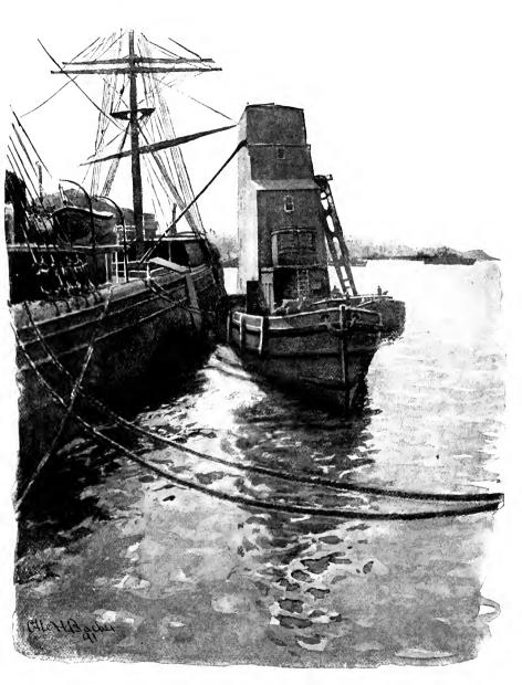
Loading Grain from a Floating Elevator.
