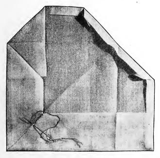
MITERED CORNERS Method of Folding and Cutting. 125
