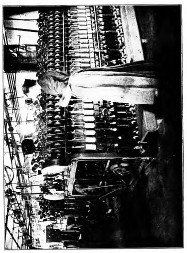
DRAWING FRAME Drawing the Roving Finer.
