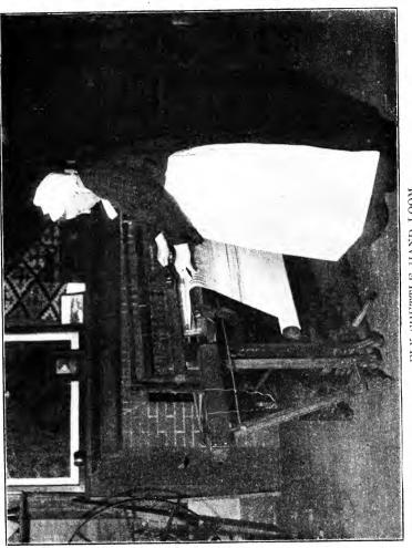
. FLY SHUTTLE HAND LOOM The Pulling of the Reed Automatically Throws the Shuttle Back and Forth and Works the Proper Time.
