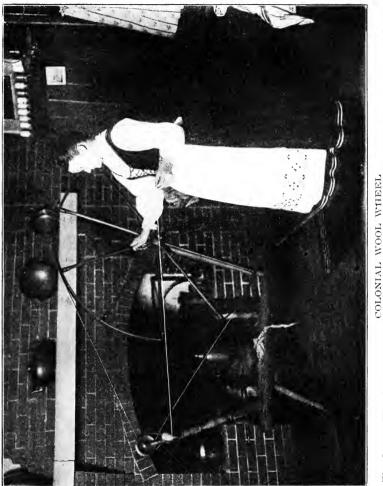
The Large Wheel Revolved by Hand Tius Turning the Spindle and Twisting the Yarn, Which Is Then Wound on the Spindle; Intermittent in Action.
