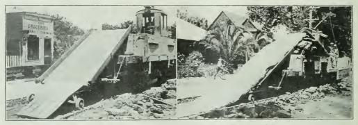
VIEWS OF MACHINE USED TO REMOVE PAVING FROM BETWEEN RAILS. Left: Ready to Begin Operations. Right: Machine in Operation.
