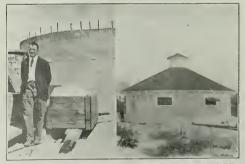
FIG. 2—PORTION OF CAISSON OF IMHOFF TANK BE-FORE LOOSENING, OCEAN BEACH, N. Y. FIG. 3—VIEW OF SUPERSTRUCTURE OF IMHOFF TANK.
