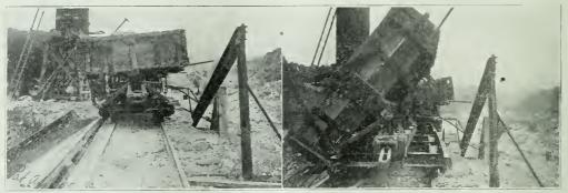
VIEWS ILLUSTRATING BEFORE AND AFTER DUMPING FOSITIONS OF INDUSTRIAL CAR, EQUIPPED WITH BRUECKER AUTOMATIC DUMPING, RIGHTING AND LOCKING APPARATUS.
