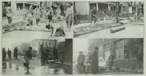
VIEWS SHOWING CONSTRUCTION PROCEDURE ON MODERN CREOSOTED WOOD BLOCK PAVEMENTS. Top Row: Pulling Strike Board on Concrete Base, Door St., To ledo-Concrete Roller in Use on Same Base. Bottom Row: Placing Pitch Cushion with Buckets and Squeegees, Superior Street Pavement, Toledo-Wood Blocks being Laid on Same Pitch Cushion.
