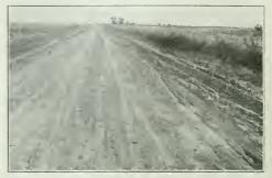
SAND-CLAY SURFACE DISCED AND DRAGGED BE-FORE FINAL DRESSING OF SHOULDERS AND DITCHES ON SAND-CLAY ROAD CONSTRUCTION—HALL COUNTY, NEBRASKA, FEDERAL AID ROAD.
