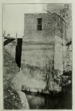
FIG. 2: CLOSE VIEW OF PENSTOCK OUTSIDE MILL SHOWN IN FIG. 1.
