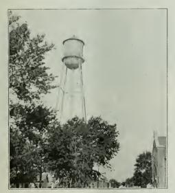
FIG. 3—THE ELEVATED STEEL TANK OF THE VIN-TON, IOWA, WATER WORKS. HEIGHT, 160 FEET; CA-PACITY, 70,000 GALLONS.
