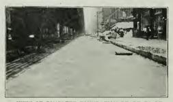
VIEW OF CONCRETE FOUNDATION READY TO RE-CEIVE GRANITE PAVING BLOCK, BOROUGH OF MAN-HATTAN, NEW YORK CITY.
