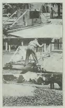
VIEWS ILLUSTRATING THE MACHINE FINISHING OF CONCRETE ROADS.
