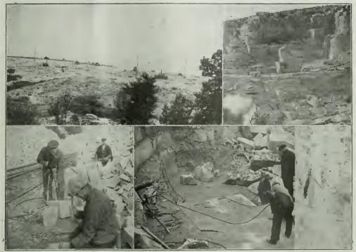
VIEWS OF QUARRYING AND CUTTING OF GRANITE PAVING BLOCKS. Top Row, Left: A Southern Quarry, a Monolithic Mass Without any Seams-Right: Northern Quarry with Bed Seams and Joint Planes. Bottom Row, Left: Cutting Elocks-Right: Breaking out Stock for Blocks.
