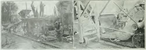
VIEWS OF PORTABLE MEASURING AND CHARGING BINS USED ON CONCRETE ROAD CONSTRUCTION ON DIALE HIGH-WAY AT FLINT, MICH., TO ELIMINATE DUMPING AND WHEELING MATERIALS ON THE SUBGRADE.
