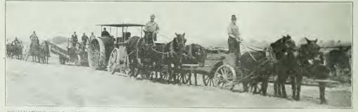
ENCAVATING AND LOADING () AY FROM RIGHT OF WAY OF CONTRIBUTARY ROAD ON SAND-CLAY ROAD CONSTRUC-TION—HALL COUNTY, NEBRASKA, FEDERAL AID ROAD.
