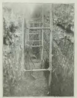
LAYING 22 IN. DRAIN TILE IN 21 FT. CUT. AT THIS DEPTH TILE ARE LAID IN CONCRETE CRADLES AS A SAFEGUARD AGAINST CRUSHING.
