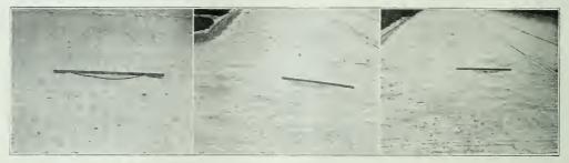
VIEWS OF BRICK PAVEMENT ON UNIVERSITY AVE., CHAMPAIGN, ILL., SHOWING HOLES WORN IN SOFT PAVING BRICK AFTER  $4\nu_2$  YEARS OF SERVICE.
