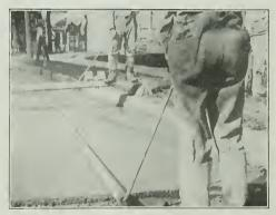
OBTAINING SMOOTH CONCRETE BASE FOR WOOD BLOCK PAVEMENT WITH SMALL ROLLER ON TEM-PLATES.
