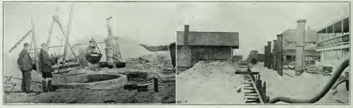
FIG. 4—PUMP WELL CAISSON IN FINAL POSITION REMOVING LAST EXCAVATED MATERIAL WITH ORANGE PEEL BUCKET WITHOUT UNWATERING CAISSON, OCEAN BEACH, N. Y., SEWERAGE WORKS. FIG. 5—VIEW SHOWS PROX-IMITY OF MAIN SEWER TO TIDAL BASIN.
