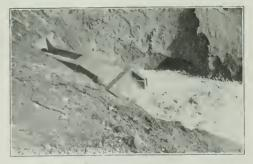
FIG. 6. VIEW SHOWING TUNNEL PORTAL, BRIDGED FLUME, DEFLECTOR AND STILLING BASIN, WITH 1,200 CU. FT. PER SECOND DISCHARGE, SIOUX FALLS SPILLWAY.
