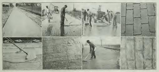
VIEWS ILLUSTRATING SEQUENCE OF OPERATIONS IN RECOMMENDED METHOD OF GROUTING A SEMI-MONO-LITHIC BRICK ROAD.
