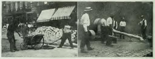
VIEWS SHOWING CONSTRUCTION OF GRANITE BLOCK PAVEMENTS IN BOROUGH OF MANHATTAN, NEW YORK CITY. Left: Applying Bituminous Filler. Right: Method of Grouting Reclipped Blocks.
