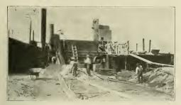
be lifted to the height it stands in the picture. Part of this frame can be seen immediately under the smoke stack. The rear end of the dryer can be lifted likewise by attaching to the bottom of the fire-box the uprights to which the rear wheels are joined. But Mr. Damewood preferred to make the small concrete piers shown, on which to rest the rear wheels, without resetting them.
