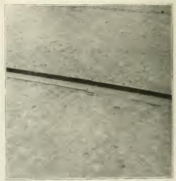
A MODERN ASPHALT FILLED GRANITE BLOCK PAVEMENT IN BALTIMORE, MD., LAID IN JULY, 1914, AND PHOTOGRAPHED IN AUGUST, 1916, NOTE AS-PHALT STILL CLINGING TO SURFACE OF BLOCKS.
