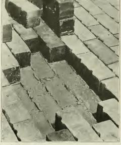
Bricks removed from rolled surface of pavement before the grout filler was applied, showing the nature of the connection between the concrete base and brick layer before the grout is applied to increase the bond between them.
