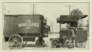
ELECTRIC DRIVEN STREET SWEEPER AND SPECIAL WAGON FOR RECEIVING SWEEPINGS TO TRANSFORT TO DUMP. WHEN IN OPERATION THE TWO UNITS ARE CONNECTED AND THE AIR PAS-SAGE, ENPS OF WHICH ARE SEEN NEAR TOP, IS CONTINUOUS.
