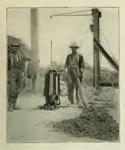
arm is then automatically locked in an upright position, to be released when the bucket is returned to the sewer and again catch the cable in its lower position. This jack is held firmly in position by being forced against the sides of the manhole with expansion screws. In manholes that are of equal size, this device can be easily and quickly removed by a pull on the chain on the shoe side.
