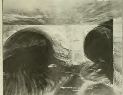
JUNCTION OF HORSE-SHOE SHAPED SEWER, ON THE LEFT, WITH A CIRCULAR SEWER, ON THE RIGHT. CONCRETE IS SPECIALLY ADAPT-ABLE TO SUCH CON-STRUCTIONS AS THIS. AS THE POSSIBILITY OF MAKING VERTICAL WALKS AND FLAT ROOFS RENDERS UN-NECESSARY THE BELL-MOUTH ABCH INTER-SECTIONS SO NECES-SARY AND SO DIFFI-CULT TO DESIGN AND CONSTRUCT IN MANY PLACES WHEN BRICK STONE IS THE OR STRUCTURAL MATERIAL USED.
