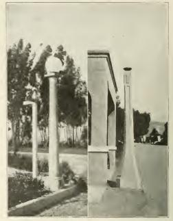
THE DESIGN OF THIS CON-CRETE POST, IN USE AT CUL-VER CITY, CAL., IS LESS DIS-TINCTIVE THAN OT HERS SHOWN, BUT STILL IS SUF-FICIENTLY DIFFERENT FROM OTHER POST DESIGNS TO BE EASILY RECOGNIZED AS INDI-VIDUAL TO THE CITY. SAN FERNANDO'S SPECIAL DESIGN IS ALSO ON GENEBAL LINES, BUT THE FLARING BASE GIVES IT AN INDIVIDU-ALITY WHICH ATTRACTS AT-TENTION, PERHAPS BECAUSE IT IS RATHER HEAVY FOR ITS PURPOSE. IT IS BUILT OF CONCRETE.
