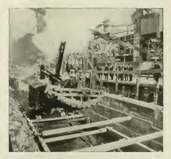
MOVING UP. THE SHOVEL LIFTING ONE OF THE PLAT-FORMS INTO PLACE. NOTE HOW FEW MEN ARE NECESSARY IN ORDER TO ACCOMPLISH THIS.
