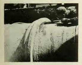
REMOVING LEAD CALKING ON 40-INCH WATER FIPE WITH OXWELD WELDING BLOWPIPE.
