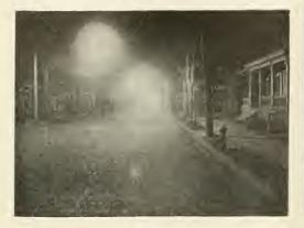
FIG. 6. NIGHT VIEW OF JERSEY AVENCE, SHOWING EYE-SUSPENSION UNITS, EQUIPTED WITH 20-IN. CONCENTRIC RE-FLECTORS, PRISMATIC REFRACTORS AND 250-C.P. EDISON MAZDA SERIES LAMPS.
