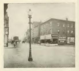
FIG. 2. DAY VIEW IN PORT JERVIS, SHOWING NOVALUX UNITS WITH 600-C.P., 20-AMP. EDISON MAZDA SERIES LAMPS.
