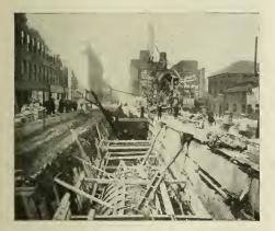
This view gives an excellent idea of the method of Mixing and transporting the concrete from a central plant. The mixed material is conveyed from the 175foot tower of Lakewood design, thru 400 feet of steel spouting, to a wooden hopper here shows, from which it is taken in concrete buggies to the sewer, into which it is dumped thru the spouting shown in the forecroup.
