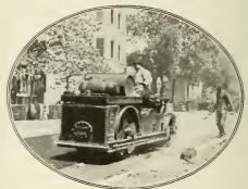
Courtesy of Popular Science Monthly. A GASOLINE MOTOR HAS ELIMINATED THE UP-RIGHT BOILER, THE STEAM AND THE NOISE OF THE STREET-ROLLER OF THE OLDER TYPES.
