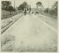
The forward end of a brick paving job on Middle Springfield Road, neur Paris, Illinois. Note steel side forms thoroly staked in place, gravel used for concrete, concrete in sacks, men filling the loading skip of the concrete mixer, bricks piled along the roadside, and wagon delivery of materials.
