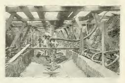
SIX NO. 2 NYE PUMPS OPERATED FROM 30-H.P. BOILEE ON SEWER JOB AT LAPORTE, IND. IN PLACES THE WATER LEVEL WAS LESS THAN ONE FOOT FROM SUFFACE. THIS WATER WAS SUCKED OUT OF THE SAND, AND WELL POINTS WERE KEPT IN OPERATION LONG ENOUGH TO ALLOW THE CON-CRETE TO SET SUFFICIENTLY TO WITHSTAND THE CROUND WATER PRESSURE. enables the Nye new model pumps to elevate a great percentage of solids to a considerable height.
