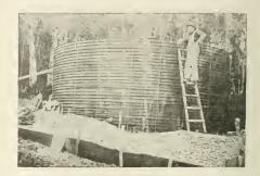
mortar. The thoro reinforcement prevents any cracking under the strains of water pressure. This new reservoir has a capacity of 25,000 gallons, and an idea of its size is given by comparison with the men standing beside it. The reservoir is used in connection with the water system of the city of Monroe, which is a center of a large farming district in Oregon. The reservoir has proven highly satisfactory, and Mr. Francis has expressed himself as highly pleased with the results.
