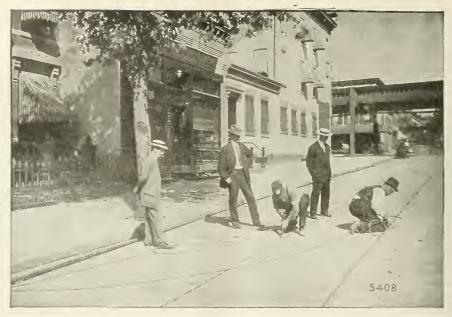
"CROWN" PICKS BEING USED TO TEAR UP ASPHALT AT 12TH STREET, BROOKLYN, N. Y.
