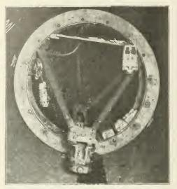
THE TESTING BULKHEAD FOR APPLYING THE PNEUMATIC TEST IN PLACE, READY FOR MAKING THE TEST.
