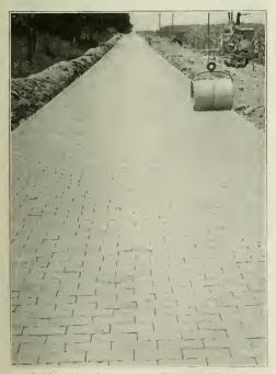
Brick surface before grout filler is applied. Note the hand roller used for rolling the brick surface; also the concrete mixer. Shoulders will be laid and compacted against the brick edges when the pavement is completed and the steel side forms are removed.
