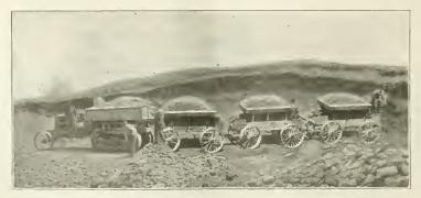
Allis-Chalmers tractor truck drawing three trailers carrying three tards of pit-run gravely weighing 3,200 pounds to the yard, and five yards in the dump body, Making a total of fourteen yards. Note the rough, rutty and sandy comdition of roadbed.
