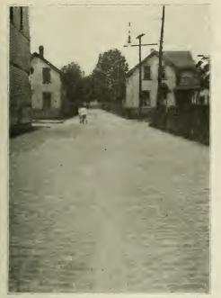
A SANITARY ALLEY PAVED WITH VITRIFIED BRICK WITH CEMENT FILLER.
