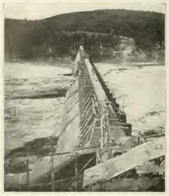
HIGHEST FLOOD EVER RECORDED. SHOWS THE AMOUNT OF WATER WHICH MIGHT PASS OVER THE COMPLETED DAMS IF THE FLOOD OCCURRED WHEN THE RESERVOIR WAS FULL. IT IS PASSING THRU A GAP IN THE UNCOMPLETED DAM.
