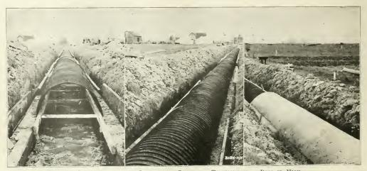
Hy-Rib archied conduit. Snyder boad, Greenfield Township, near Detroit, Mich. Hy-Rib in place with inside and Hy-Rib in place with outside Comleted conce outside forms for walls, forms for starting concrete lay-
