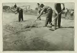
II. CLEANING OFF THE DIRT AND LOOSE STONE DOWN TO THE SOLID BASE.
