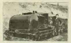
Bell locomotive of 24-inch oage, 6-ton weight, hauling gravel on highway construction work.
