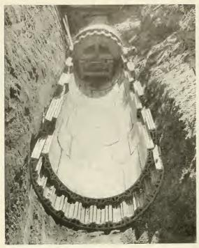
IV. A 48-INCH SEGMENTAL BLOCK SEWER UNDER CONSTRUCTION IN WAUSAU, WIS.
