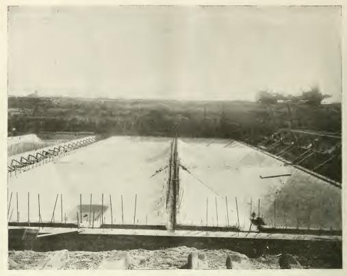
ROCHENTER SEWAGE DISPOSAL PLANT. SHOWING SLOPING TANK BOTTOMS WHERE RATHER DRY MIXTURE HAD TO BE USED, WATERPROOFED WITH TRUSS-CON WATERPROOFING PASTE, CONCENTRATED, C. ABTHUR POOLE, SUPERVISING ENGINEER.
