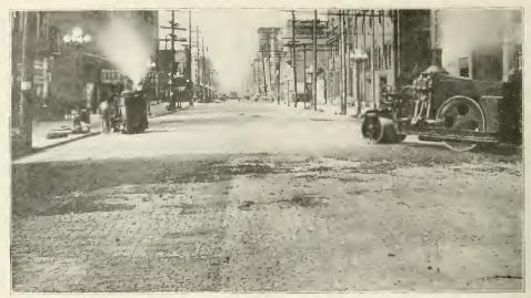
RESURFACING OLD BRICK PAVEMENT WITH ASPHALT USING BINDER COAT AND WEARING SUR-FACE COAT. ASPHALT LAID FROM CURB TO CURB.
