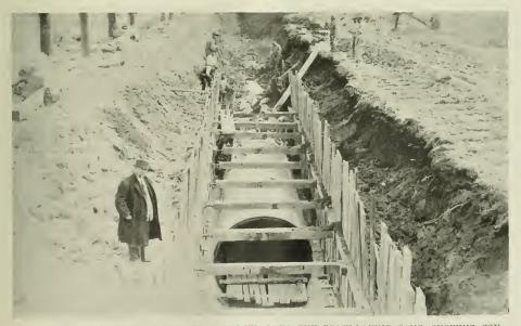
LOOKING BACK FROM THE STEAM SHOVEL OVER THE BRICK-LAVING GANG, SHOWING COM-PLETED INVERT IN FOREGROUND, ARCH FORMS, BRACING AND SHEETING IN PLACE, BRICK LAY-ERS AT WORK AND FIRST STAGE OF TRENCH-FILLING FROCESS.
