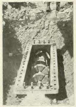
MACHINE FOR CLEANING WATER MAINS IN PLACE IN SPECIAL BOX CONSTRUCTED IN THE MAIN FOR THE PURPOSE OF INSERTING AND RE-MOVING THE CLEANING MACHINE. A COVER IS BOLTED TO THE BOX WITH A WATER-TIGHT JOINT.
