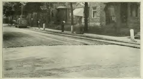
RESURFACING OLD BRICK PAVEMENT WITH ASPHALT, USING BINDER COAT AND WEARING SUR-FACE COAT. NEW BRICK GUTTERS AND ASPHALT LAID BETWEEN THEM.
