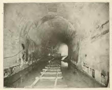
A SECTION OF MILL CREEK SEWER, ST. LOUIS, MO., WHERE THE SEWER HAS A SEMI-CIRCULAR ARCH, VERTICAL SIDE-WALLS AND AN INVERT WHICH IS ALMOST FLAT. STEEL FORMS SEEM TO HAVE BEEN USED IN THIS CASE. THE WATER STANDING ON THE BOTTOM MAKES IT DIFFICULT TO SEE THE DESIGN AS IT REALLY IS. THIS SECTION OF THE SEW-ER IS A ROCK TUNNEL LINED WITH CONCRETE WHICH WAS PLACED BY COMPRESSED AIR.
