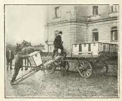
OCHNNER SYSTEM OF REMOVAL OF REFUSE AND STREET SWEEPINGS. NOTE STRICTLY SANITARY CONDITIONS AND FA-CILITIES FOR LOADING CANS BY SMALL TRUCK ON INCLINED RAILWAY.
