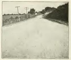
VI. THE COMPLETED FIBERED ASPHALT SURFACE ON AN OLD TELFORD-MACADAM BASE.
