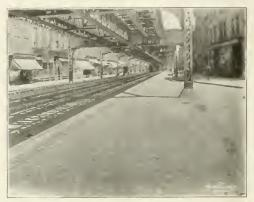
THE COMPLETED PAVEMENT ON SUNDAY. COMPARE JOINTS AND SURFACE OF THE NEW PAVEMENT LAID UNDER THE LATEST IMPROVED SPECIFICATIONS WITH OLD GRANITE BLOCKS IN THE STREET CAB TRACKS LAID SEVERAL YEARS ACD UNDER THE OLD SPECIFICATIONS.
