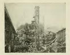
RANSOME - CANNIFF PNEUMATIC MIXER AND PLACER WITH A SPOUTING SYSTEM IN BRIDGE CON-STRUCTION.
