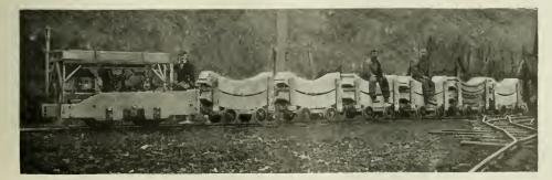
part way in the tunnel, where the blocks are then picked up by a compressed air locomotive, which operates in the tunnel and out to the work. At the present time this is about two miles out from shore.
