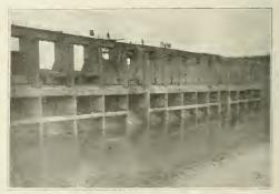
THE UPPER SIDE OF THE COMPLETED DAM. THE FLOOD GATES ARE SHOWN PART RAISED AND PART LOWERED. THEY OPEN AUTOMATICALLY WHEN THE FLOOD REACHES A CERTAIN HEIGHT. THE BRIDGE BETWEEN THE PIERS SUSTAINING THE GATE IS SHOWN ABOVE EXTREME HIGH WATER.
