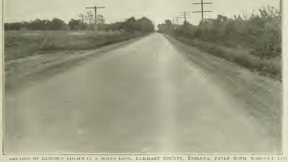
SECTION OF LINCOLN FIGURATED MILES LONG, ELKHART COUNTY, INDIANA, PAVED WITH WHE-CLT LUG BRICK IN 1915; PHOTOGRAPHED A YEAR LATER. BRICK PORTION 16 FEET WIDE BETWEEN 6-INCH CURBS, OR EDG-INGS. CEMENT-GROUT FILLER USED.
