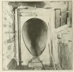
AN EGG-SHAPED SEWER LAID ALONGSIDE THE SUBWAY CONSTRUCTION IN SEVENTH AVENUE, MANHAITAN BORO XEW YORK CITY, OF REINFORCED MONOLITHIC CONCRETE. THE MASSIVE CHARACTER OF THE STRUCTURE AND THE ELAB-ORATE PROVISIONS FOR A WATER-TIGHT JOINT WHEN THE SEVER IS EXTENDED ARE CLEARLY SHOWN IN THE PHOTO-CRAPH, ALSO THE NATURE OF THE FOUNDATION CONSTRUCTED FOR IT. WOODEN LAGGING WAS EVIDENTLY USED IN THE FORMS.
