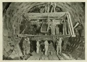
ceeded 21 pounds to the square inch, altho it is expected that It will be necessary to increase this to 25 or 27 pounds when maximum depth under the harbor is reached at approximately 60 feet below the surface of low tide.
