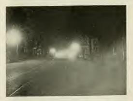
FIG. 5. NIGHT VIEW OF PIKE STREET, SHOWING NOVA-LUX ORNAMENTAL UNITS EQUIPPED WITH 600-C.P., 20-AMP, EDISON MAZDA SERIES LAMPS.
