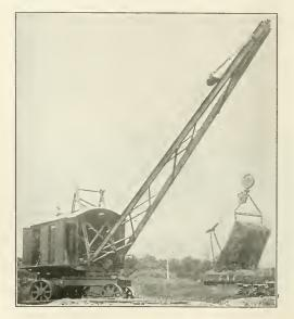
ternal steel sprockets and chain from back axle. The front axle suspension is three point for traveling. The upper frame is rigidly held in position by jack nuts when working. The back, or driving, axle is a solid steel forging. The front axle is built up of 12-inch I-beams with stub ends for removing in case of wear.
