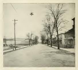
FIG. 3. DAY VIEW IN PORT JERVIS, SHOWING AN EVE-SUSPENSION UNIT WITH 20-IN. CONCENTBIC REFLECTOR, PRIS-MATIC REFRACTOR, AND 250-C.P. EDISON MAZDA SERIES LAMP.
