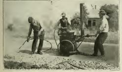
ROAD OILER WITH HEATER AND HAND PUMP.
