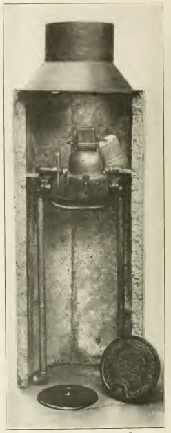
METER BOX AS INSTALLED IN 15-IN. TILE. THE SURFACE OF THE GROUND COMES FLUSH WITH THE TOP OF THE COVER. THE TOP, SHOWN LYING FLAT ON THE GROUND, IS FOR FROST PROTECTION, AND THE ONE STANDING IS THE LOCKED TOP COVER.
