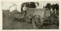
2.7 miles per hour can be attained on high gear, and 2.1 miles on low. The machine can be turned either backward or forward within a 15-foot circumference.
