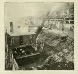
NOTE THE HEAVILY CONSTRUCTED PLATFORMS OF FLOATS ON WHICH THE SHOVEL IS OPERATED. THESE PLATFORMS, AS MAY BE SEEN, ARE SHAPED TO THE EDITOM CONTOUR OF THE TRENCH. SEE ALSO THE NEXT PHOTOGRAPH.
