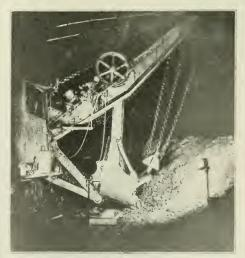
We are illustrating a type of Milburn portable light on night excavation. This type, as illustrated, burns 10 hours on a charge without attention. Still another type is designed for attachment on large mechanical equipment. The reflector is fastened to the boom, front housing or other point from which work is illuminated, while the generator is placed in the operator's cab, connection being made with a hose.
