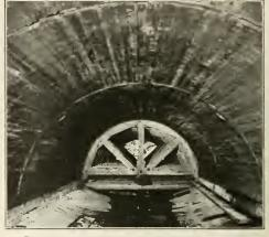
CIRCULAR ARCH AND INVERT WITH DIFFERENT RADII AND A LOW VERTICAL WALL RETWEEN, AS USED IN NEW YORK. FORMS WITH WOODEN RIBS, BRACES AND LAGGING WERE USED IN THIS CONSTRUCTION.
