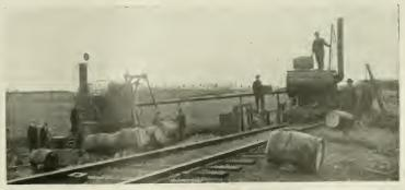
BOGIE IN POSITION AFTER TIP-PING STONE INTO KOEHRING MIXER LOADING BUCKET.
