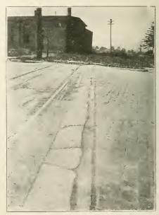
HEAVY STONE HEADER AND BACKING AT DIAGONAL END OF BRICK PAVEMENT ALONG RAILROAD TRACK, NECESSARY TO PREVENT MOVEMENT FROM EXPANSION.
