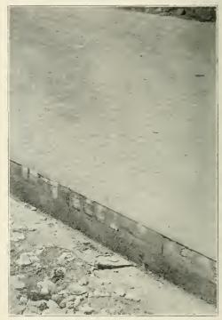
The edge of the monolithic brick pavement, showing concrete base and intimate connection of base and brick layers. A gravel and earth shoulder will be compacted against this vertical surface, which requires no curb.
