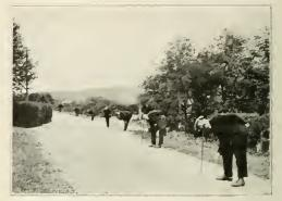
STETHOSCOPES IN USE TO TRACE MOTION OF CLEANING MACHINE THRU THE PIPE. AS THE MA-CHINE PASSES EACH MAN HE WALKS QUICKLY TO THE OTHER END OF THE LINE OF OBSERVERS SO THAT THE LINE OF MEN ROLLS ALONG THE ROAD AT SAME RATE THAT THE MACHINE TRAVELS.
