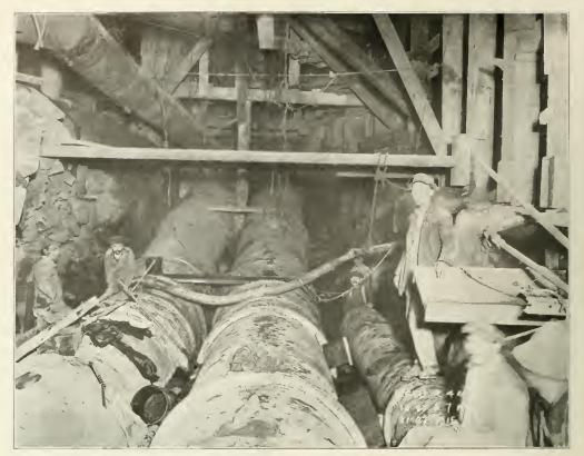
INVERTED SEWER SIPHONS OF CAST-IRON USED IN CARRY-ING SEWERS UNDER THE SUBWAY IN NEW YORK SUBWAY CONSTRUCTION. THE TWO LARCE PIPES ARE FIVE-FOOT STORM SEWERS. THE SMALLER PIPE IS A 24-INCH SEWER TO CARRY THE DRY-WEATHER FLOW OF SEWAGE. NOTE THE SPECIALS AT THE BEND AT THE LOWEST POINT IN THE SIPHON.
