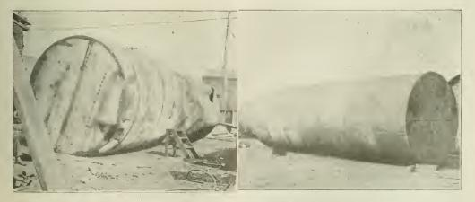
"BEFORE" AND "AFTER" PHOTOS OF TEXAS OIL COMPANY TANKS RESTORED TO USE WITH BOXER HAMMERS.
