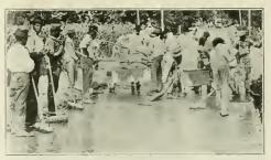
Spreading the first coat of the grout filler for joints. Note the brooms for sweeping the grout into the joints. The concrete mixer and brick-laying gang in the background show how closely the finishing follows the beginning of the pavement laying.
