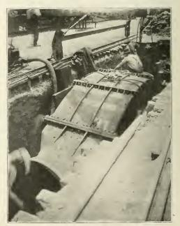
A CAST-IRON SEWER CONNECTION OF LARGE SIZE.
