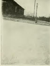
TWO ROWS OF BRICK REPLACED OVER ELECTRIC LIGHT WIRE TO STREET LAMP.
