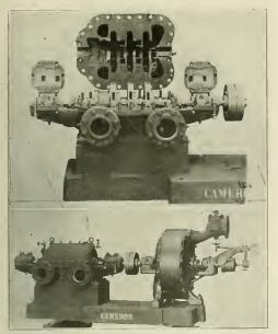
ABOVE: THREE-STAGE BOILER-FEED PUMP, SHOWING INTERNAL CONSTRUCTION AND ACCESSI-BILITY OF PARTS.
