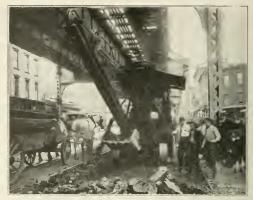
KEYSTONE STEAM SHOVEL ENCAVATING OLD WEARING SUBFACE AND DUMPING INTO WAGON. NOTE CLOSE QUARTERS IN WHICH MACHINE WORKS AND ITS ADAPTABILITY TO THE PECULIAR CON-DITIONS.
