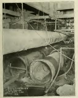
Two CAST-IRON STORM SEWERS BELOW, EACH FIVE FEET IN DIAMETER. TEMPORARY STEEL PIPE FLUME ABOVE TO CARRY SEWAGE OURING CONSTRUCTION OF THE INVERTED SIPHONS UNDER CONSTRUCTION BELOW.
