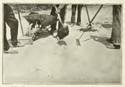
IV. TAMPING FIBERED ASPHALT MIXTURE INTO THE DEEPER DEPRESSIONS IN THE ROAD SURFACE,
