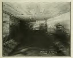
A DESIGN USED IN NEW YORK INVOLVING A CHRCULAR IN-VERT WITH LARGE RADU'S, VERTICAL SIDE-WALLS AND FLAT SLAB TOP, THE CLEAR MARKS OF BOARDS AND NAILS SHOW THAT WOODEN FORMS WERE USED HERE ALSO.
