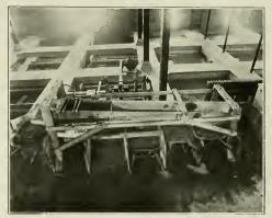
TROUGH WITH SCREENS FOR WASHING AND SCREENING GRAVEL FOR USE IN WATER FILTERS OF GRAND RAPIDS, MICH., WATER WORKS. NOTE SIX SIZES OF SCREENED GRAVEL AND SAND.
