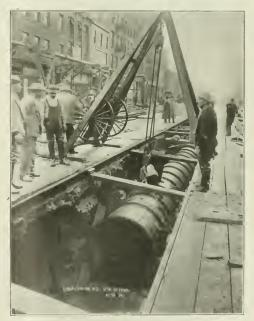
A FIVE-FOOT RIVETED STEEL SEWER FOR TEMPORARY USE IN CONNECTION WITH NEW YORK SUBWAY WORK. AN A-FRAME DERRICK, AS DESCRIBED IN THE ARTICLE, HANDLES TURNE PIPES.
