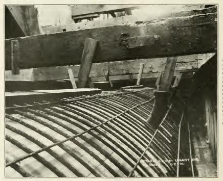
OUTSIDE OF FORMS USED IN CONSTRUCT-THE ING SEWER SHOWN IN THE PRE-CEDING PHOTOGRAPHS. SHOWING THE WOODEN LAGGING. THE DE-BAR REIN-FORMED FORCEMENT. CIRCUM-FERENTIAL AND LONG-ITUDINAL, THE METH-OD OF HOLDING HOUSE-CONNECTION PIPES IN PLACE UNTIL CONCRETE IS POURED AND SET. AND THE TRENCH BRACING.
