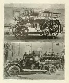
quirements. Only slight and inexpensive changes were necessary to make the old bodies conform closely to the new motor truck chassis.
