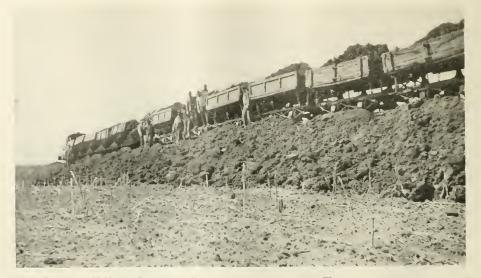
AT THE DUMP. ONE OF THE MCMILLAN CONTRACTING COMPANY'S TRAINS OF FOUR-YARD WESTERN CARS MAKING A FILL IN THE CON-STRUCTION OF MEYER BOULEVARD, KANSAS CITY.
