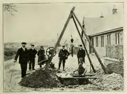
THE PILE ON THE LEFT SHOWS THE AMOUNT OF MATERIAL, TUBERCULATION, SCRAPED FROM 6,000 FEET OF 14-INCH MAIN. THE COVER OF THE BOX FOR INSERTING THE MACHINE IN THE LINE IS SEEN SUPPORTED OVER THE HOLE DUG DOWN TO THE BOX.
