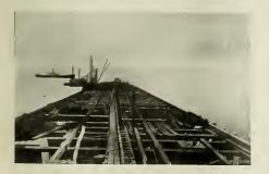
DISCHARGE PIPE FROM A RANSOME-CANNIFF PLACER CONVEYING CONCRETE FOR CONSTRUCTION OF A COAL PIER, PIPE LAID IN CENTER OF FALSE WORK.
