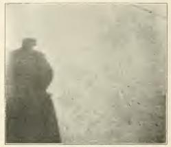
LARGE IRREGULAR PATCH IN GROUT FILLED BRICK PAVEMENT. SURFACE PRACTICALLY RE-STORED TO ORIGINAL SMOOTHNESS AND CONTIN-UITY.
