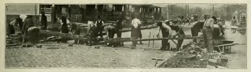
depth of about an inch greater than the required finished depth. At the same time it is thoroly spaded and joggled in order to compact the concrete and to bring only mortar in contact with the side forms.
