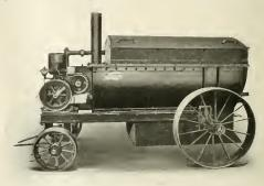
large-sized fire-box underneath, adapted for hurning wood, coal or coke. The tank is jacketed by a heating chamber, which is extended on the front so as to receive and enclose a Kinney pump, which is driven by gasoline engine, as shown in the cut, or may be driven hy hand power, as desired. The important advantage of the heating chamber is that the pump is kept heated at all times, thus preventing the hardening of material within the pump and so preventing its operation.
