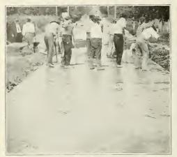
Applying the second coat of coment filler, which leaves the surface smooth and the joints full. Note the squeegees used in spreading this coat.
