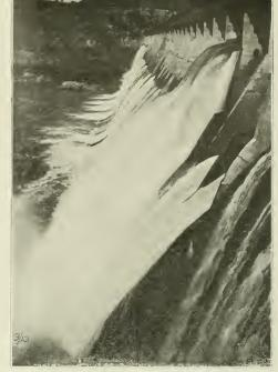
WATER FLOWING OVER DAM WITH FLOOD GATES CLOSED, BEING THE NORMAL CONDITION. ONE OF THE FLOOD GATES IN THE FOREGROUND IS OPEN TO SHOW THE EFFECT UPON THE FLOW OF WATER. IF ALL WERE OPEN THE RESERVOIR WOULD SOON BE DRAWN DOWN TO THE LEVEL OF THE CREST OF THE DAM.
