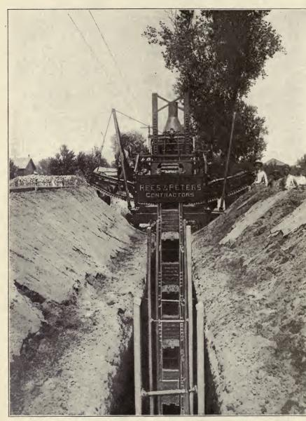
PARSONS TRENCH EXCAVATOR CUTTING A 15-FOOT DITCH IN A 14<sup>1</sup>/<sub>2</sub>-FOOT ALLEY Courtesy of G. N. Parsons Company, Newton, Iowa
