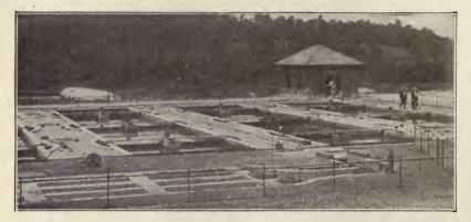
Fig. 51. Installation of Imhoff Tanks at Atlanta, Georgia
