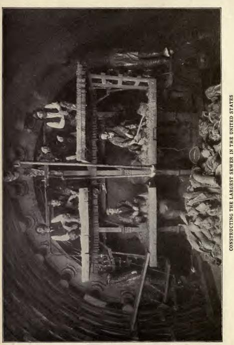
View of men at work in tunneling shield; wooden forms also shown. Sewer lined with brick laid in "Utica" hydraulic cement. View of 39th Street intercepting sewer, Chicago, 111.
