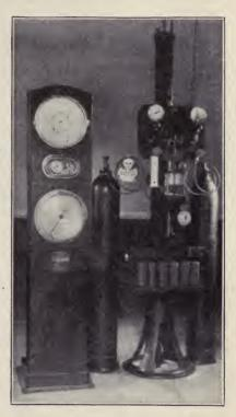
Fig. 70. Automatic Control Apparatus for Liquid Chlorine
