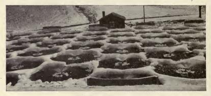
Fig. 61. Danville, Pennsylvania, Sprinkling Filters in Operation at 14 Degrees below Zero
