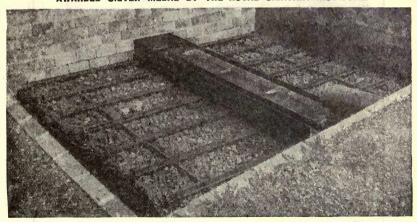
Tipping Apparatus and Distributor for Sewage Trickling Filter. Sewage Lifts, Valves, Penstocks, &c.
