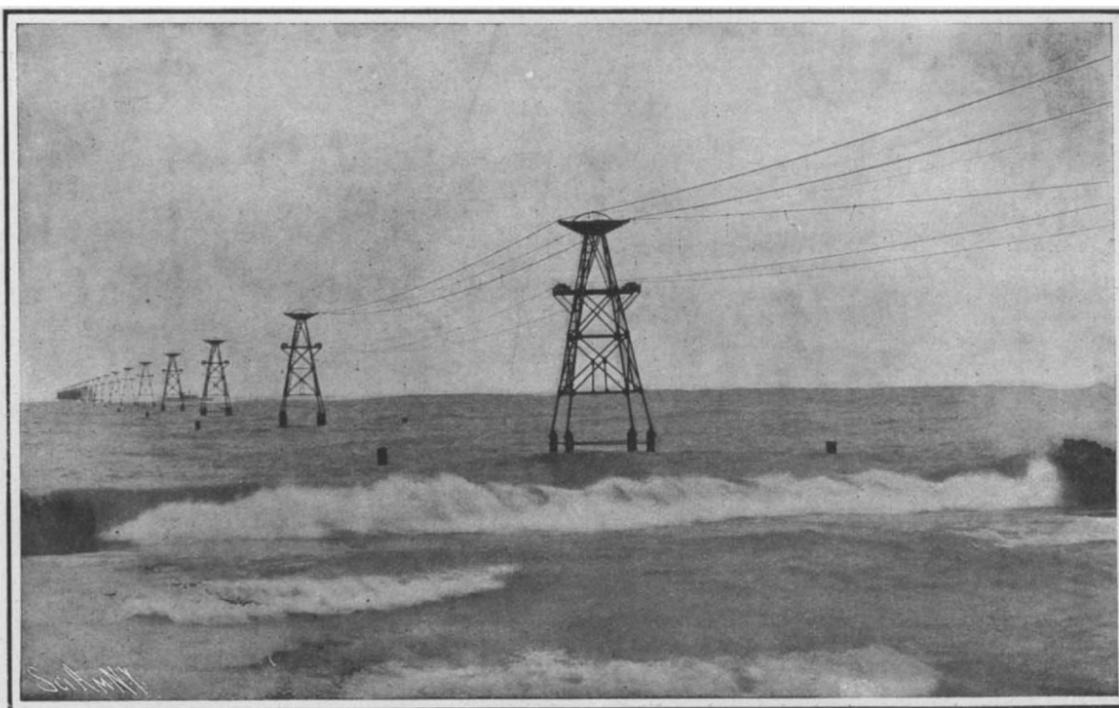
The Cableway Stretching Out Over the Lake for a Distance of 8,000 Feet.
