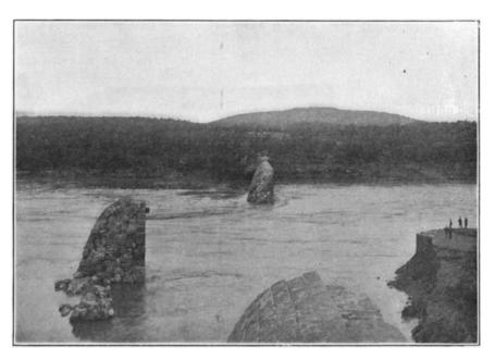
The Break Viewed from the Headgate Masonry, Showing Section of Dam Moved Bodily Downstream.
