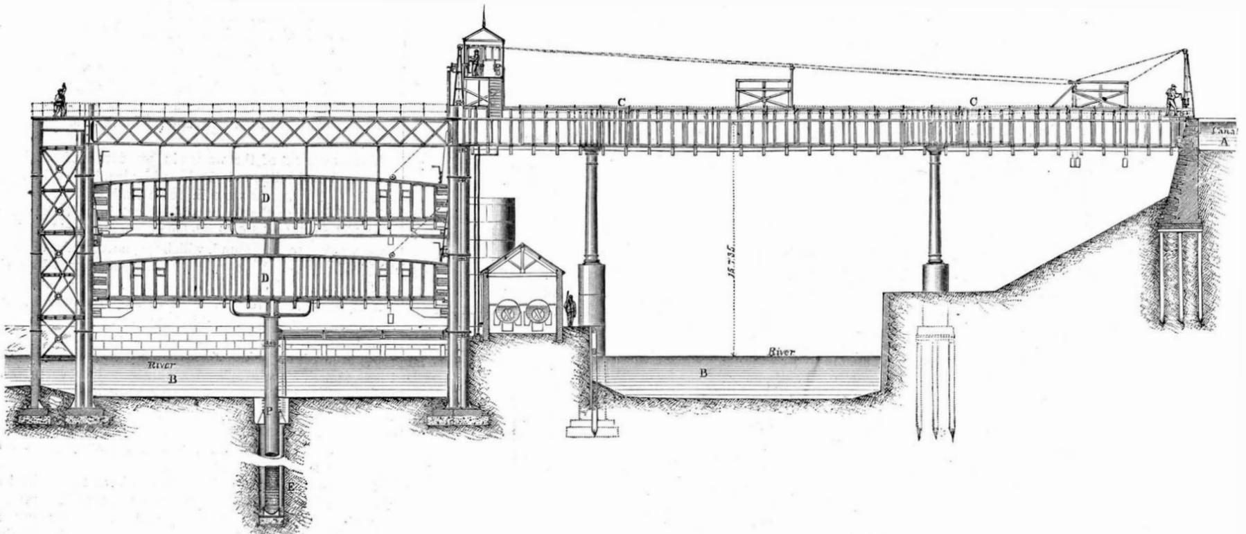
HYDRAULIC ELEVATOR FOR CANAL BOATS.—CONSTRUCTED IN THE WEAVER AT AUDERTON, ENGLAND.
