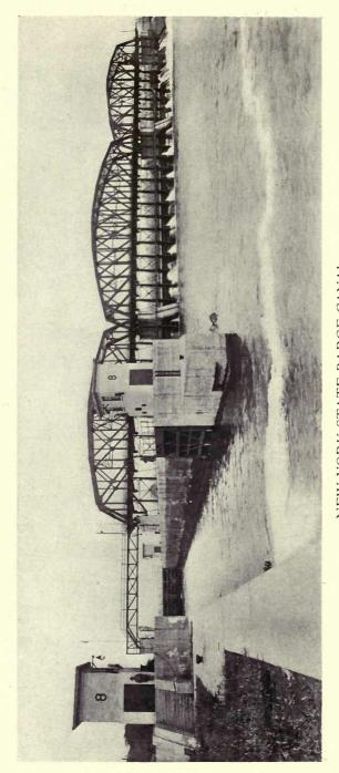
Movable dam and lock in Erie Branch View showing gates down, and the structure fulfilling its purpose as a dam Courtesy of State Engineer and Surveyor's Dept. NEW YORK STATE BARGE CANAL
