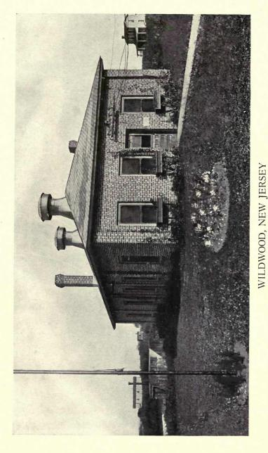
General view of R-W sewage treatment plant. Process consists of mechanical fine screens with direct discharge of the effluent into the bay
