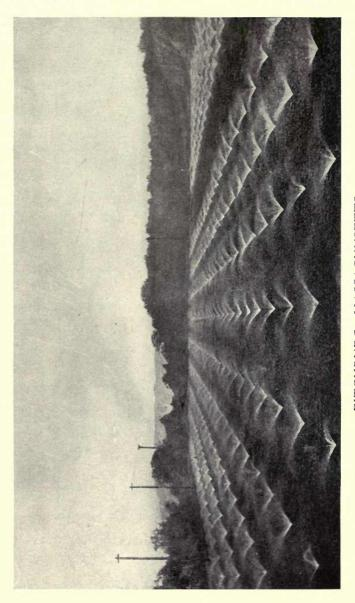
FITCHBURG, MASSACHUSETTS Trickling filter plant in operation
