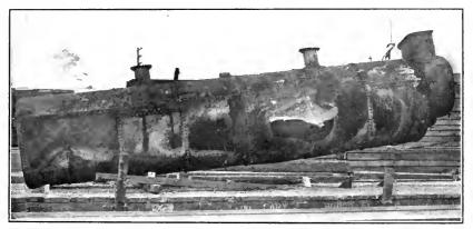
BOILER BURNED AND RUPTURED AS A RESULT OF LOW WATER. The Blow-Off on This Boiler Was Found Open When the Deeris Was Being Cleared Away After the Accident.
