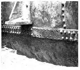
A DEFECTIVE BUTT STRAP DISCOVERED BY INSPECTION.
