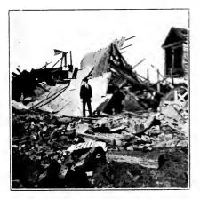
One man was killed, two were injured and the ginning plant of Clark and McCowan, near Florence, S. C., was demolished by a boiler explosion on September 20, 1921. The boiler had been idle for six months and during this time had been repaired by welding on a patch about 14" x 24", the work being done by the oxy-acetylene process. When the boiler was put into service it exploded, the failure having its origin at the welded patch. The boiler was blown into the air and landed about 350 yards away.
