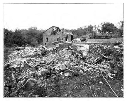
UNFAMILIARITY WITH THE PROPER ADJUSTMENT OF SAFETY VALVES CAUSED THIS BOILER EXPLOSION.
