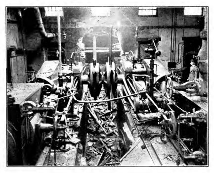
FLYWHEEL EXPLOSION AT A FIBRE MILL.
