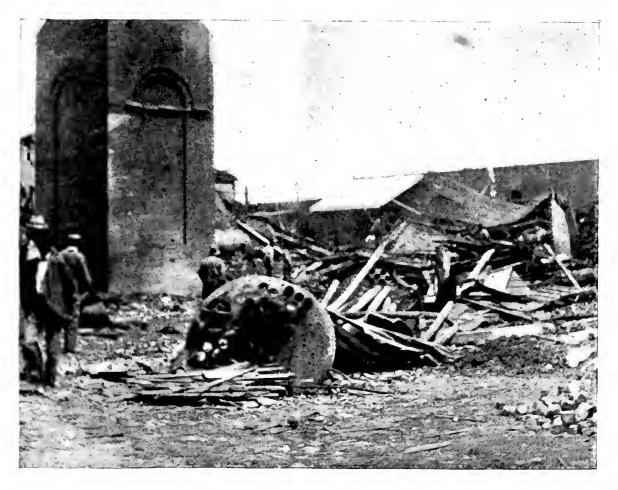
FIG. 3. - SHOWING THE EXPLODED BOILER.
