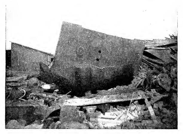
FIG. 2.- Snowing the Shell of the Bursted Boller.
