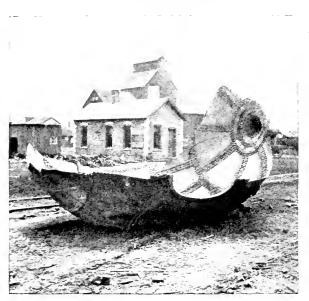
FIG. 2.— AN EXPLODED ROTARY.
