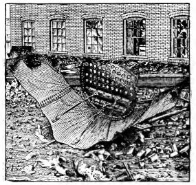
FIG. 3.—THE REAR END OF THE BOILER.
