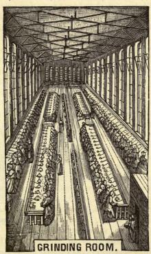
160 girls are busily employed cross and straight grinding steel pens on wood cylinders covered with emery. The room in which the finished pens are placed in boxes measures 54 by 30 feet, and in it alone are employed
