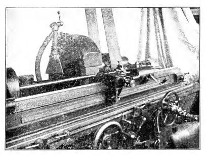
Fig. 329. Norton Grinder with 5 $\frac{1}{2}$ -Inch Face Wheel for Grinding Ford Axles and Drive Shafts
