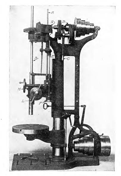
Fig. 175. Standard Power Feed Driller Courtesy of Reed-Prentice Company, Worcester, Massachusetts
