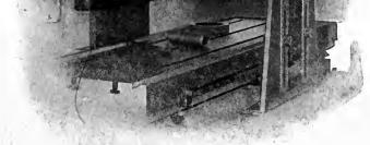
Fig. 229. Vertical Milling Head Attached to Horizontal Milling Machine Courtesy of Brown and Sharpe Manufacturing Company, Providence, Rhode Island
