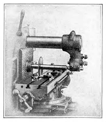
Fig. 198. Sawing Flat Stock Courtesy of Brown and Sharpe Manufacturing Company, Providence, Rhode Island
