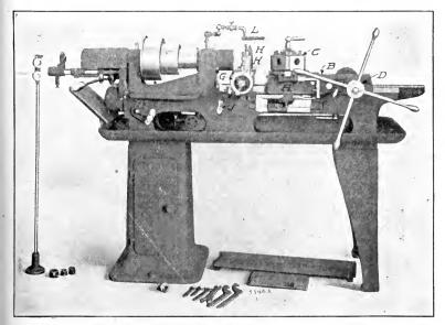
I ig. 295. Turret Lathe, Hand-Revolved and Hand-Fed Courtesy of Pratt and Whitney Company, Hartford, Connecticut
