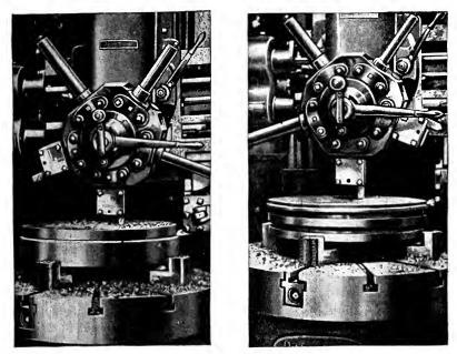
Fig. 354. Three Views of Bullard Turret Lathe in Action On Piece Shown, Time Required for Setting Tools, Turning, Chamfering, Boring, and Finishing, 80 Minutes.
