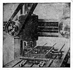
Fig. 228. End Milling Attachment on Planer
