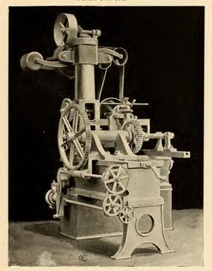
GEAR-CUTTING AND WHEEL-DIVIDING MACHINE.
