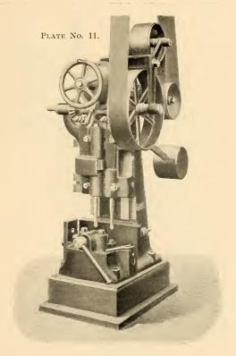
TWO-SPINDLE RAIL DRILLING MACHINE.
