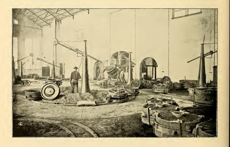
VIEW IN CAR-WHEEL FOUNDRY OF PENNSYLVANIA RAILROAD, SHOWING HYDRAULIC MOULDING CRANES AND LADLE-TILTING DEVICE.
