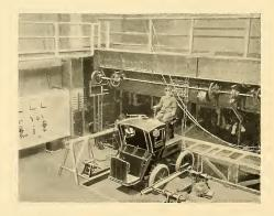
8-TON TRAVELLING CRANE.—FOR HANDLING STORAGE BATTERIES IN THE POWER HOUSE OF THE ELETCRIC VEHICLE CO., NEW YORK.
