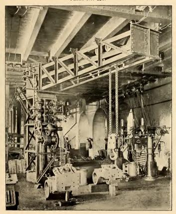
6-TON ELECTRIC COLUMN JIB-CRANE.
