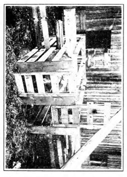
On top of the panel notched in  $\beta_4$  inch is a 2-inch strip passing parallel with the gates, but over the panels. This strip stops the gates from falling inward. As
