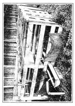
panels; third space, water trough, 4 inches deep, 8 inches wide; fourth space, 8-inch board notched 1 inch at each cross section of panel. The panel has a 6-inch
