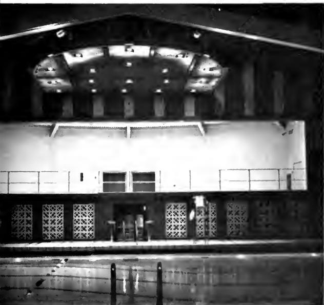
Hershey's new outdoor-indoor pool. Two southern quadrants of wall roof section are movable. Two 2-horsepower, two-speed gear motors drive each section. It takes approximately
