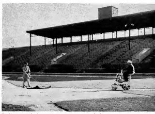
Rolling and dragging are a part of the routine care and maintenance important for any type of infield.
