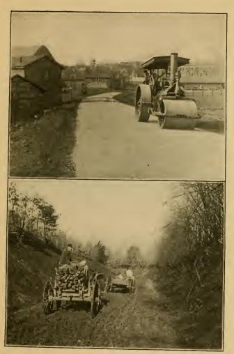
Fig. 70. Jefferson Memorial Road, from Charlottesville to Monticello, Va., as it is and as it will be. The upper view shows a sample section, improved with the equipment brought by the U. S. Good Roads train, in April, 1902.
