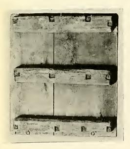
13. Wooden Mould for Making a Stove Plate.
