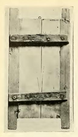
Wooden Mould for Making the End Plate of a Five- or Six-Plate Stove.
