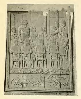
IO. Wooden Mould for Making a Stove Plate.
