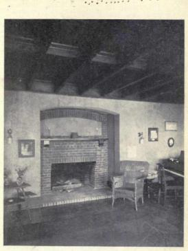
A simple and exceedingly effective recessed design in brick and rough plaster. The hearth is raised above the floor
