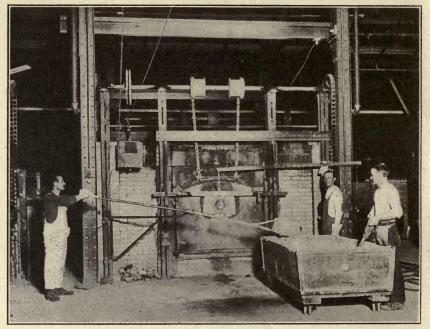
FIG. 25.—Batch about to be filled by means of long "scoop" into glass-nelting pot inside the furnace. (Photograph by J. Harper Snapp at the Bausch & Lomb Optical Co.)
