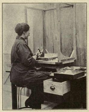
FIG. 52.—Trimming defects from pressed plates of optical glass. (Photograph by J. Harper Snapp at plant of Spencer Lens Co.)
