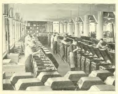
Fig. 39. In this room the mechanical parts of the phonographs are finally adjusted to make the complete machine
