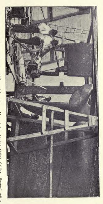
using the author's equipment. out removing the rudder from the vessel. The welding of this rudder was accomplished on August 10, 1905, The above is a photograph taken while welding the rudder of the United States Collier "Brutus"
