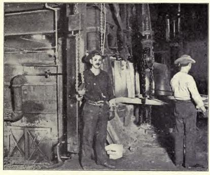
A large coal-fired forging furnace changed to oil fuel by simply building a combustion chamber of proper form and proportions in the former fire-box and placing a burner at the end of this combustion chamber. With this slight change the operator has now an oil furnace wherein the fire is under perfect control and from which he obtains a maximum quantity of output of superior quality.
