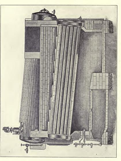
Fig. 7. Equipment of Heine Boiler-High Setting.
