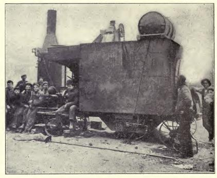
Portable Asphalt Mixer equipped with oil burner.
