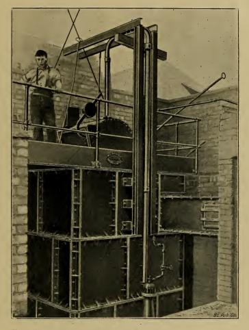
FIG. 45.—PERSPECTIVE VIEW SHOWING EXTERIOR OF MASON'S REFUSE GASIFER.
