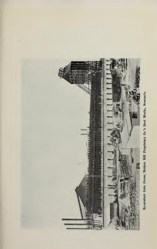
The charge per oven is 7.9 tons of crushed coal, the burning period twentyfour hours, and the loss from breeze (small coke) and burnt coke is  $2\frac{1}{2}$  per cent. By-products are recovered, the generated gases being used for lighting and heating, and the tar sold to a separate company for further treatment. A complete plant for the preparation of sulphate of ammonia has been installed, and is producing a salt of excellent quality.
