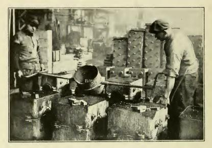
FIG. 3. A BULL LADLE IN USE. (The handle is provided with a swivel, and one man tilts the ladle while the other man simply sustains a part of the weight.)
