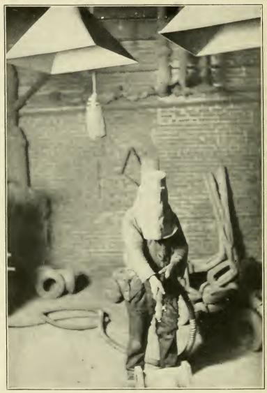
FIG. 15. A SPECIAL CHAMBER FOR SAND-BLASTING. (Strong air suction, through the exhaust hoods shown in the upper part of the picture, will remove a large quantity of the dust that is created, but it would be better if the ducts were placed in the floor, with gratings over them, or in the side walls. The helmet which the operator is wearing is of a type commonly used in work of this kind. As explained in the text, no entirely satisfactory helmet has yet been devised.)
