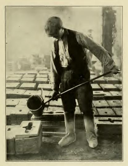
FIG. 4. POURING FROM A HAND LADLE.
