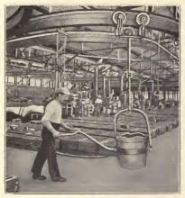
Fig. 140. Overhead Track and Trolley.
