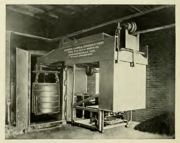
FIG. 231.—CHARGING THE CUPOLA WITH A DROP BOTTOM BUCKET, OPERATED ELECTRICALLY.
