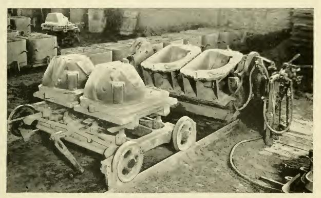
FIG. 170.—Two Drags Molded on Molding Machine.
