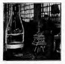
Fig. 85. Making Cores on a Small Jolt Machine.
