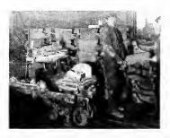
Fig. 122. Placing the Flask Around the Pattern.
