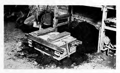
Fig. 158. The Drag Flask is Placed on and Clamped, Ready for Rolling Over.
