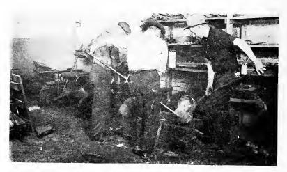
Fig. 165. Pouring Must Take Place Rapidly Due to the Thin Sections.
