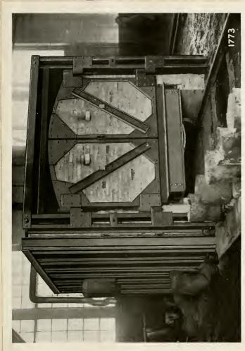
OIL-RURNING ANNEALING OVEN IN CONVERTER STEEL FOUNDRY OF DELAWARE & HUDSON CO, WATERVLIET, NEW YORK CAPACITY: 5 TO 10 TONS
