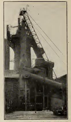
ENTERIOR VIEW OF BLAST FURNACE. SHOWING PIPES FOR CONVEYING WASTE GASES TO STOVES, DUST SEPARATOR IN FOREGROUND.
