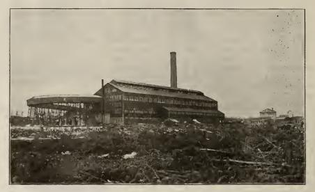
GENERAL VIEW OF THE COMPLETED PLANT AT CONISTON. NOTE THE CURVED LINE OF TRESTLES CARRYING THE TRACKS THAT RUN UNDER THE ORE BINS AND ON THE CHARGING FLOOR LEVEL.
