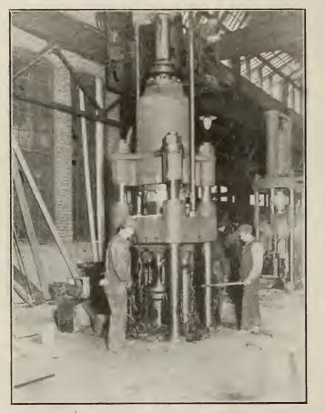
FIG. C-350-TON R. D. WOOD HYDRAULIC PRESS PERFORM-ING FIRST OPERATION ON 18-POUNDER SHELL FORGINGS.
