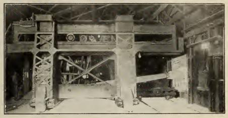
CHARGING MACHINE DEPOSITING MATERIAL IN FURNACE.
