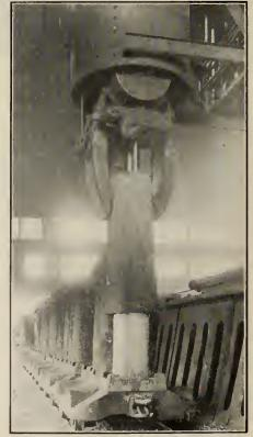
STRIPPING THE MOULD FROM THE HOT INGOT.
