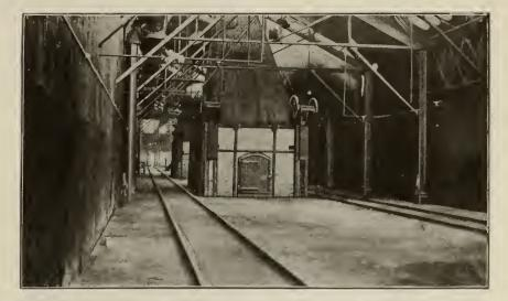
CHARGING FLOOR, SHOWING TOP OF A FURNACE.
