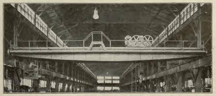
TRAVELLING CRANE EQUIPPED WITH PLATFORM AND HANDRAILINGS.
