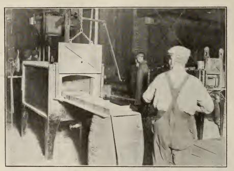
FIG. E—BELLEVUE ANNEALING FURNACES FOR HEAT TREATING STEEL SHELL FORGINGS IMMEDIATELY THEY LEAVE THE WOOD PRESSES.
