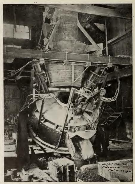
SHOWING POURING POSITION OF ELECTRIC FURNACE, AND VENT THROUGH WHICH ESCAPING GASES ENTER THE SUSPENDED STACK; MOFFAT-IRVING SMELTERS, LTD., TORONTO.
