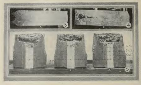
Fig. 3. Ingot made by "Hadfield" process; perfectly sound, free from blow holes, piping and segregati n. Fig. 4. Ingot made in ordinary manner; unsound, having blow holes, piping and segregation. Fig. 5. Upper portions of three ingots made by the "Hadfield" process.
