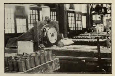
FIG. 12. FIFTH DRAW OF AN 18-PDR. SHRAPNEL SHELL CARTRIDGE CASE ON A "BERTRAM" PLANER.
