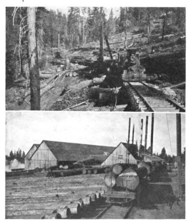
Figure 64. Logging in California. Powerful steam engines pull the logs from the woods to the railroad and load them on flat cars. Photo by the author.
