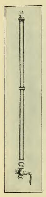
Fig. 13.—Bamboo spray rod. (Quaintance and Siegler.)
