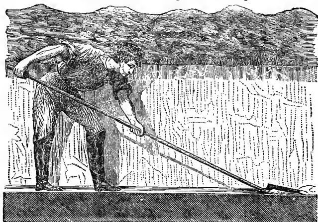
Fig. 36.—Position of Workman and Use of Finishing Scoop.
