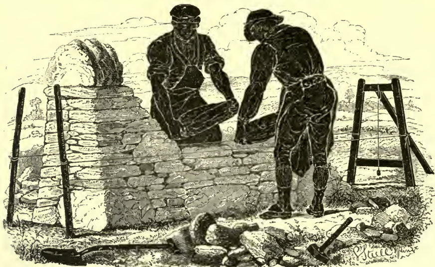
THE BUILDING A DRY-STONE DYKE.
