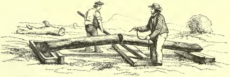
PREPARATION OF THE TIMBER FOR BOUCHERIE'S METHOD OF PRESERVING IT.
