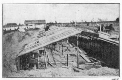
FIG. 16.—A storage house in process of construction. Note the method used of placing ventilators in the roof.
