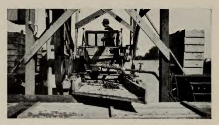
Fig. 1.—Hinged basket type dipper, showing spraying and spreading apron.
