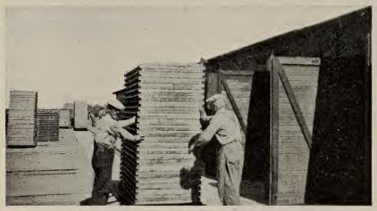
Fig. 4.-Loading a truck of trays into the dehydrater.
